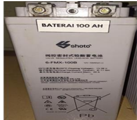
Figure 2.4 100 Ah Battery Solar Power Plant Off-Grid 450 V
