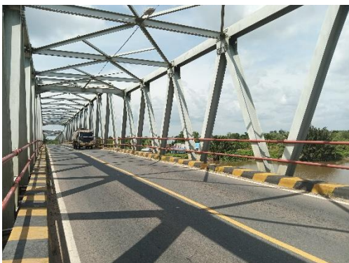
Figure 3. Overview of Pawan 2 Bridge
