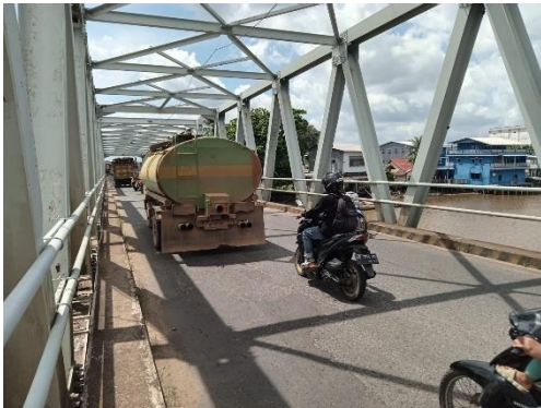
Figure 1. Overview of Pawan 1 Bridge
